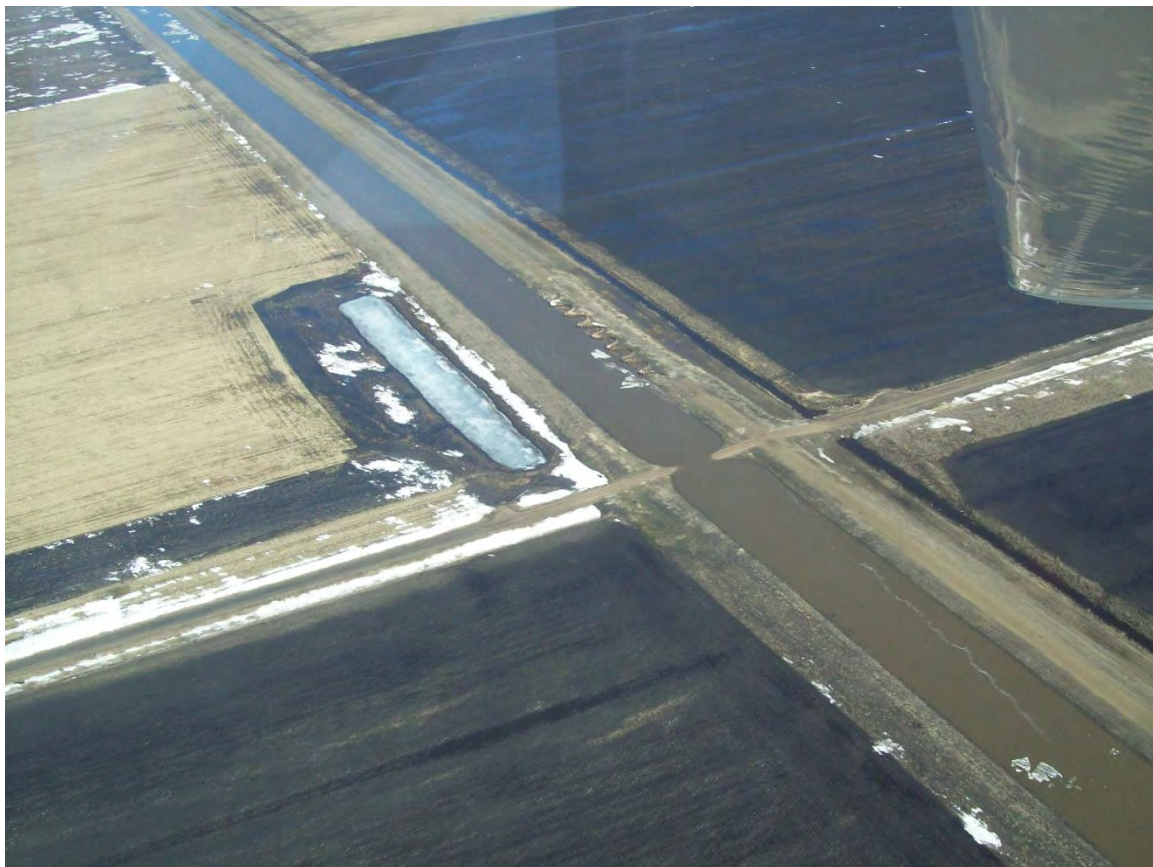
North Ottawa Impoundment Emergency Spillway.
